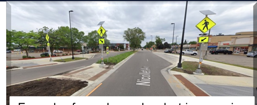
Example of an enhanced pedestrian crossing
